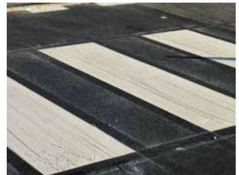
QMS installed 18,000m<sup>2</sup> of QMS HyperGrip™ across the 69 sites highlighted for works within the project and treated a total of 66 manhole covers with the **PREMARK® Anti-Skid** material. The works were a combination of day and night working to minimise disruption to the road user and maximise operative safety and saw the work completed in 97 shifts.
