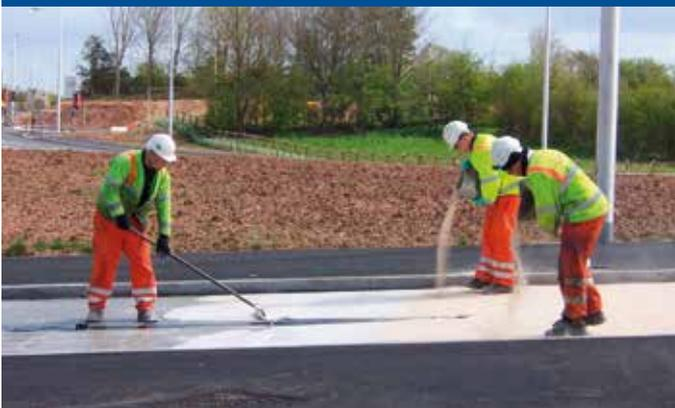
Full cure of the QMS HyperGrip™ system is achieved within one hour, allowing the site to be fully swept of loose aggregate before opening to the public.
