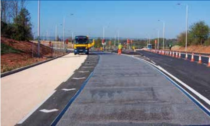
The QMS HyperGrip™ system for the contract required a scratchcoat void filler to be installed prior to the installation of the surface course. This was to ensure that the surface voids within the new bituminous substrates did not compromise the aesthetic appearance and the functionality of the finished system. The scratchcoat void filler material is applied to the surface via a flat bladed squeegee and allowed to cure.
