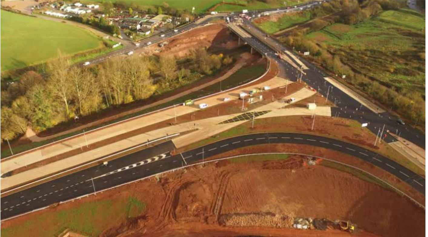
The newly constructed South Devon Link Road is a 5.5km dual carriageway built to bypass the existing A380 between Newton Abbot and Torbay to ease congestion through the village of Kingskerswell and to improve the connection of Torbay into the Highway Infrastructure, paving the way for an improved local economy. First proposed over 50 years ago, the project was granted full approval in May 2012 with work beginning in the autumn of that year.
