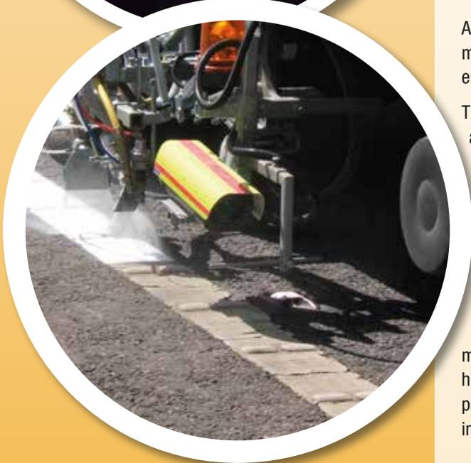
Achieving outputs of 30,000lm per shift this speed of application results in up to 75% reduction in traffic management costs, increased safety by less time spent on the network and benefiting motorists by cutting delays due to maintenance.
